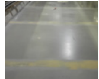
Here lightweight floor panels were bonded to metal frames using 3M™ Scotch-Weld™ Epoxy Adhesive DP125. The adhesive’s low viscosity offered excellent self-levelling properties with strong adhesion to GRP.
